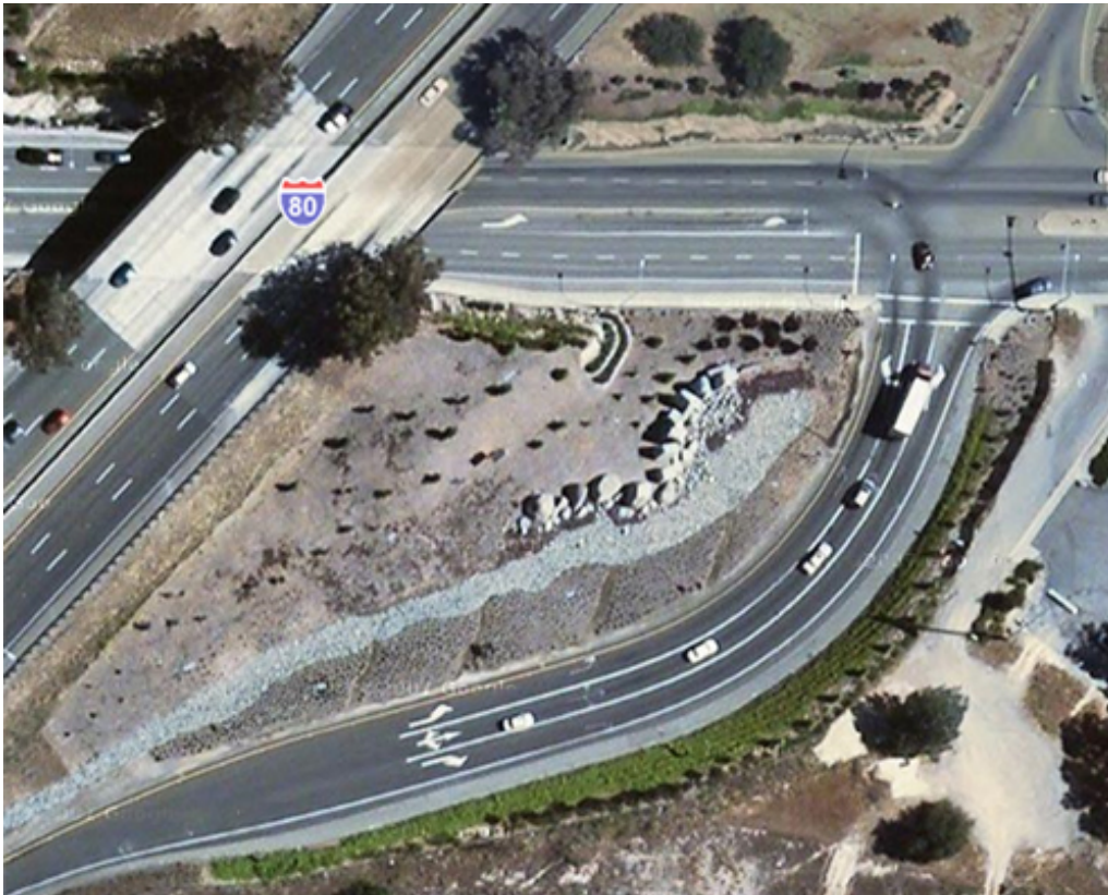
View from across the off-ramp looking toward the sign and Interstate 80. Images courtesy of Kristin Posehn.
